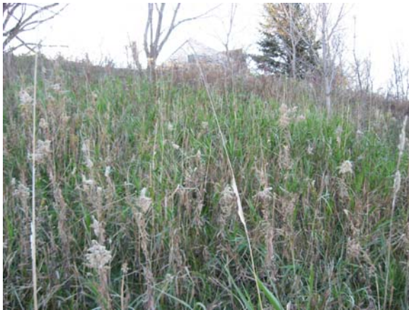
Road cut slope, NE end Phase II
